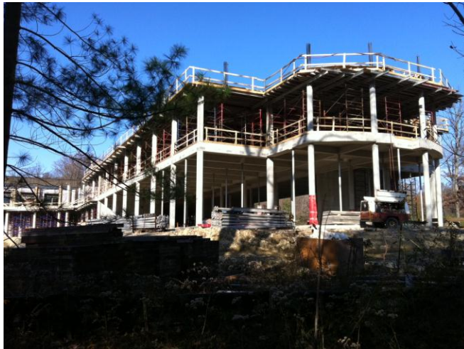
New Academic Wing Under Construction
